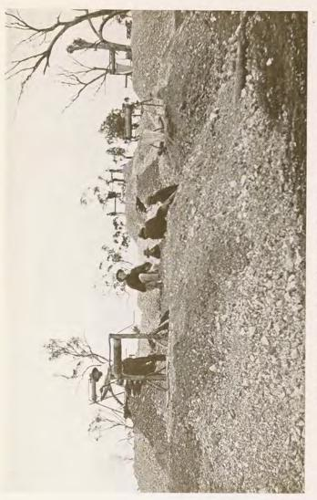
Where 60 feet of hard siliceous rock has to be pierced before the opal strata is met with. WORKINGS AT THE THREE-MILE, LIGHTNING RIDGE,
